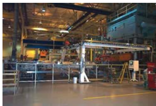
One of two QPF cells at GM's New Hudson, MI, plant.
